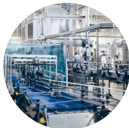
Industrial Water Systems
