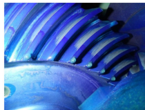
Gear Contact Inspection
