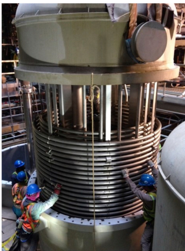
Chemical—Tank & Agitator Installation
