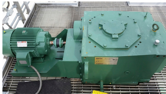
Lightnin CMX prior to commissioning
